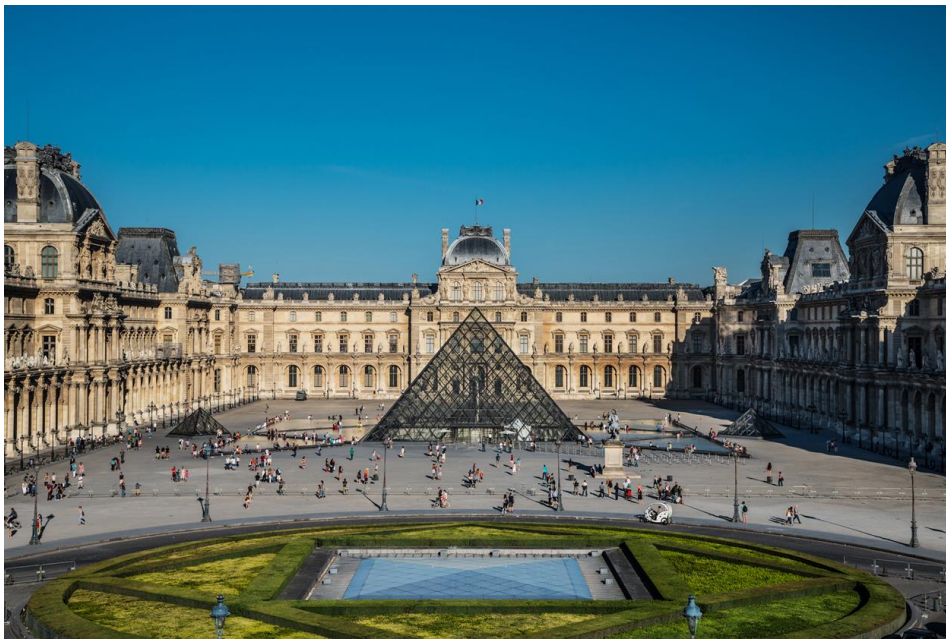
Grand Louvre Modernization (1993), Paris
