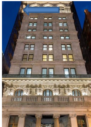
108 Leonard is also known as the Tribeca clock tower building. EVAN JOSEPH PHOTOGRAPHY
